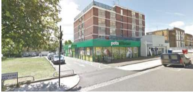
Flats above former garage: Richard Seifert architect, 1965
