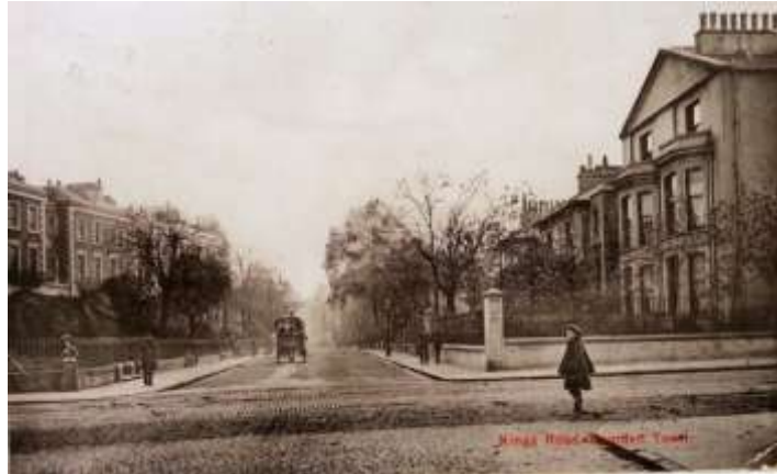
Postcard of 'Kings Road and Camden Road' to northwest- Brecknock Crescent left and Camden Cottages right
