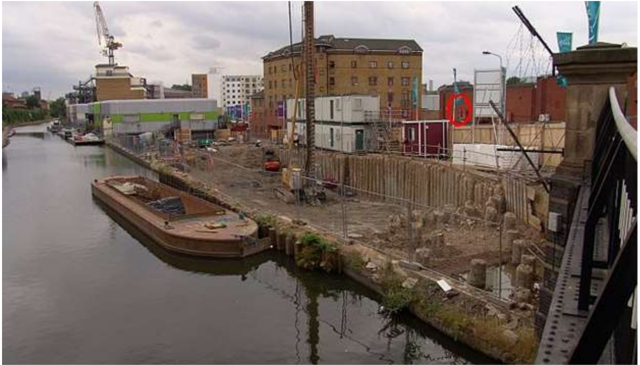
Camden Wharf – photo 6 2006 during construction of foundations for a housing block
