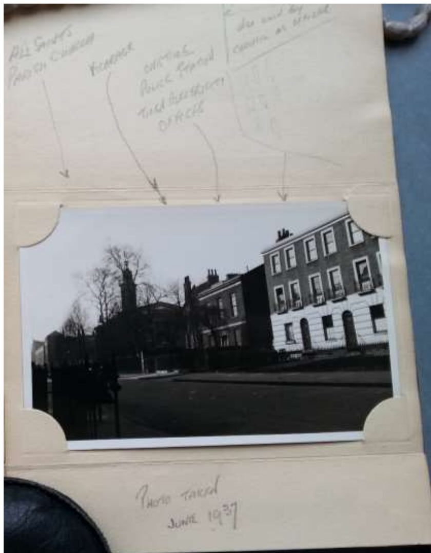
LMA/4278/01/005. Saint Pancras Electric Lighting. W.H. Barnes' photograph of 57 Pratt Street.
